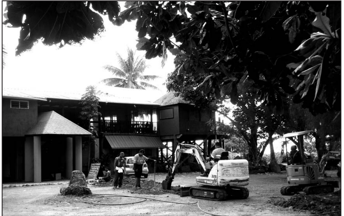
Trenching outside Staircase Restaurant
