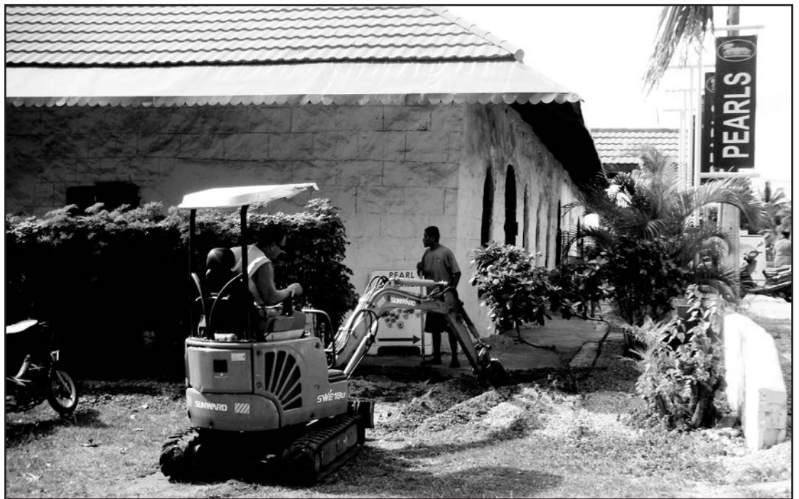
Trenching service line outside Beachcomber
